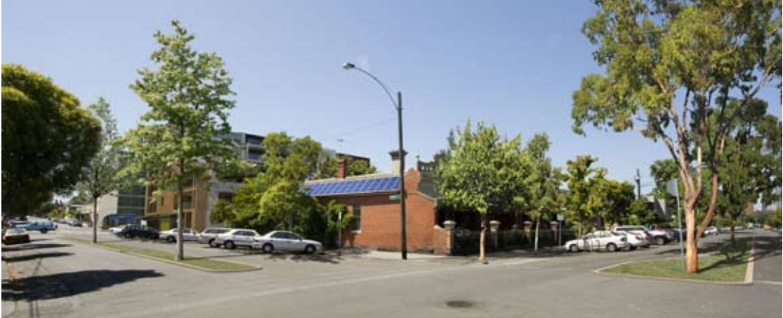
After (demonstrates the minimising of the impact of the corridor development on the streets behind)
