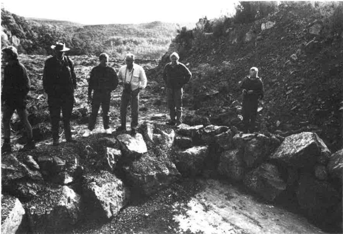
ACKMA members consider the rehabilitation work – Conference '95.
