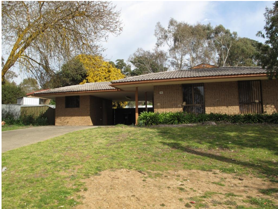
Accommodation, Inverbrackie alternative place of detention, July 2011.
