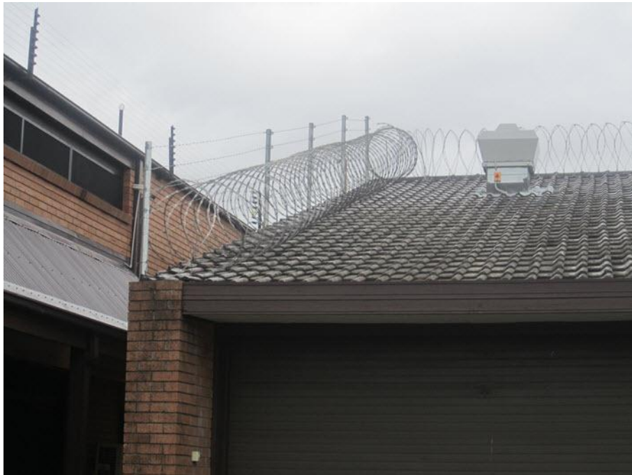
Blaxland compound, Villawood IDC, February 2011.
