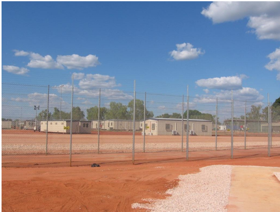
Looking into Curtin IDC through perimeter fence, May 2011.
