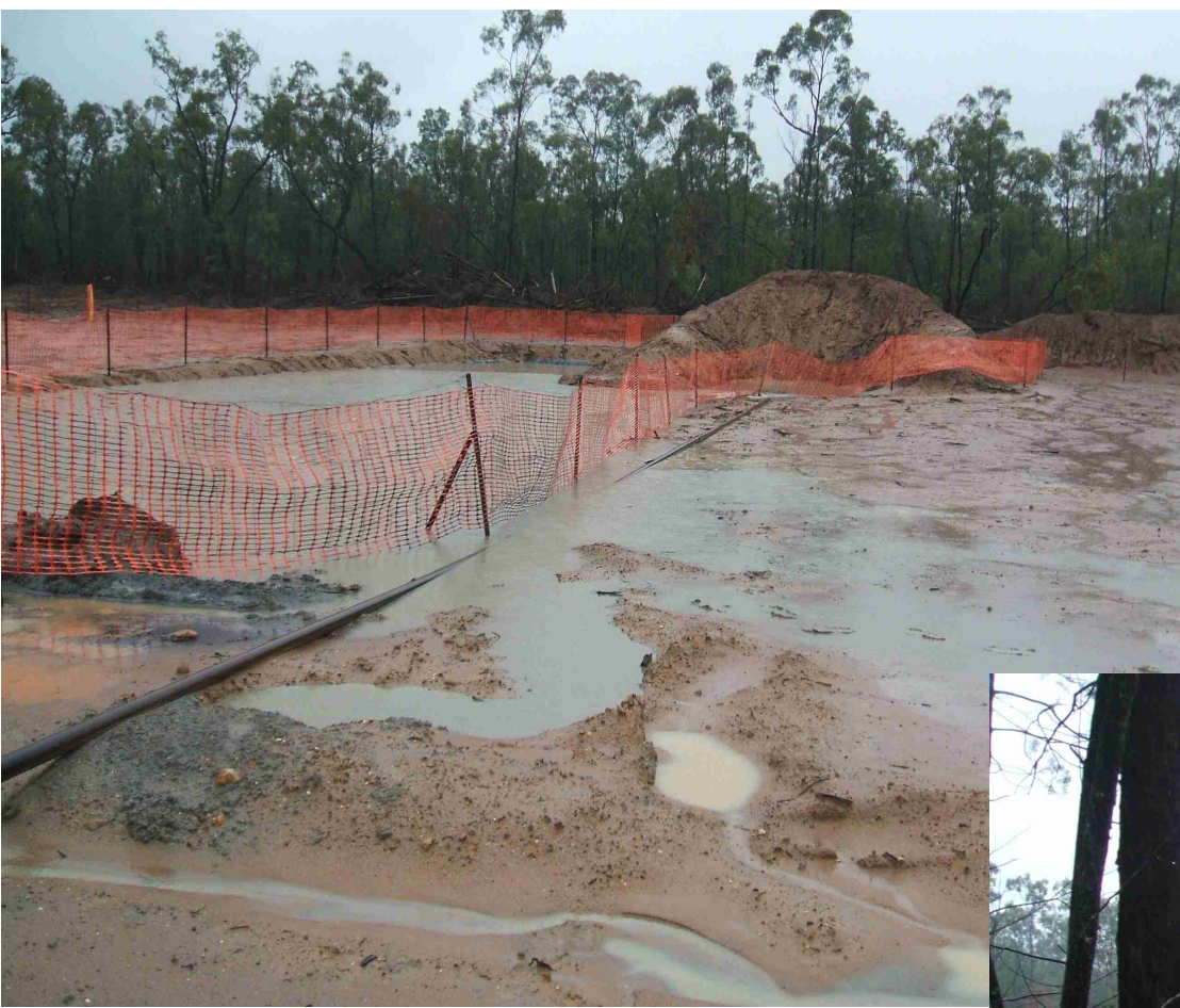
Photo 10. Dewhurst 16H, exploratory corehole. Unlined drill pond overflowing on private land during rain event in the Pilliga. Taken 2010.
