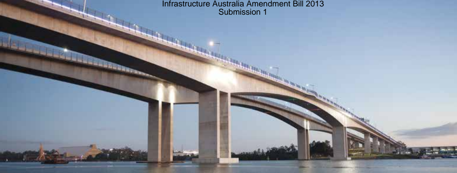
Gateway Bridge, Brisbane
