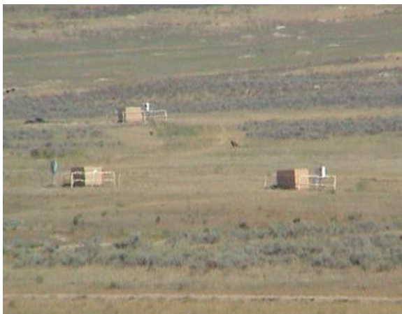
CBM Wells Constructed as Part of a Well Pod in Montana
