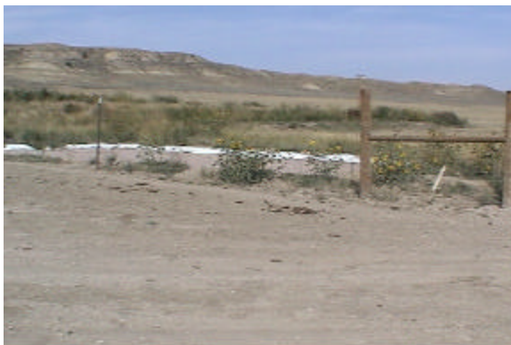
Constructed Wetland for the Treatment of Produced Water in Wyoming
