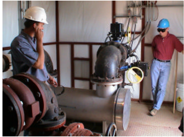
Ultra-Violet Sterilization Treatment Of CBM Produced Water
