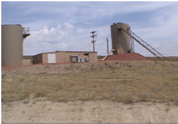
Deep Injection Facility for the Disposal CBM Produced Water, Wyoming
