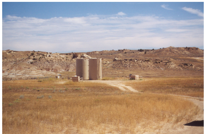
Photograph of typical CBM wells co-located with injection well, Wyoming
