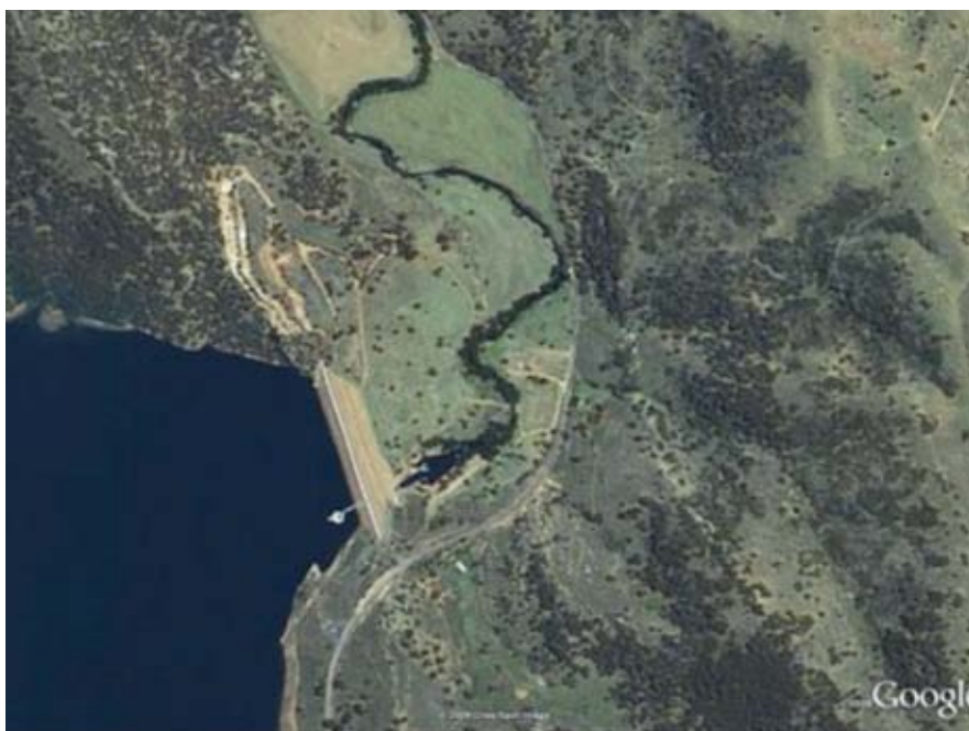
Plate 5: Peel River immediately downstream of Chaffey Dam (Foster 2003).
