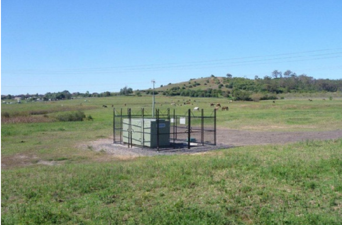
Figure 4: enclosed well in Western Sydney area
