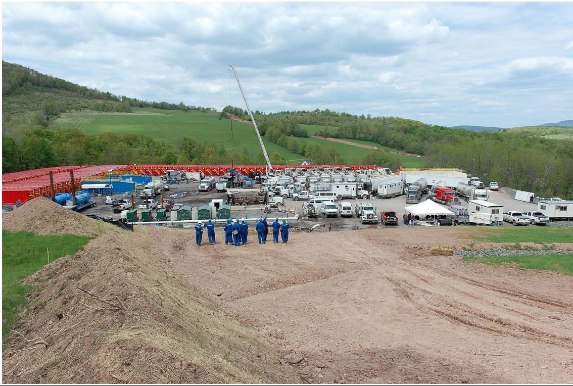
Photo 6_2 - A representative view of completion activities at a recently constructed well pad, showing a newly created access road in foreground (New August 2011)
