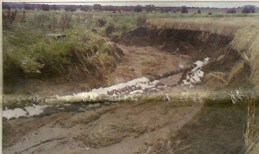
The Central Ranges gas pipeline exposure on Peter and Charmaine Cook's farm, north of Coolah.
