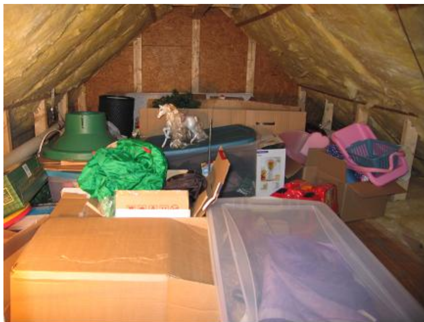
Figure 4-6: Photograph of the furnished attic space interior.
