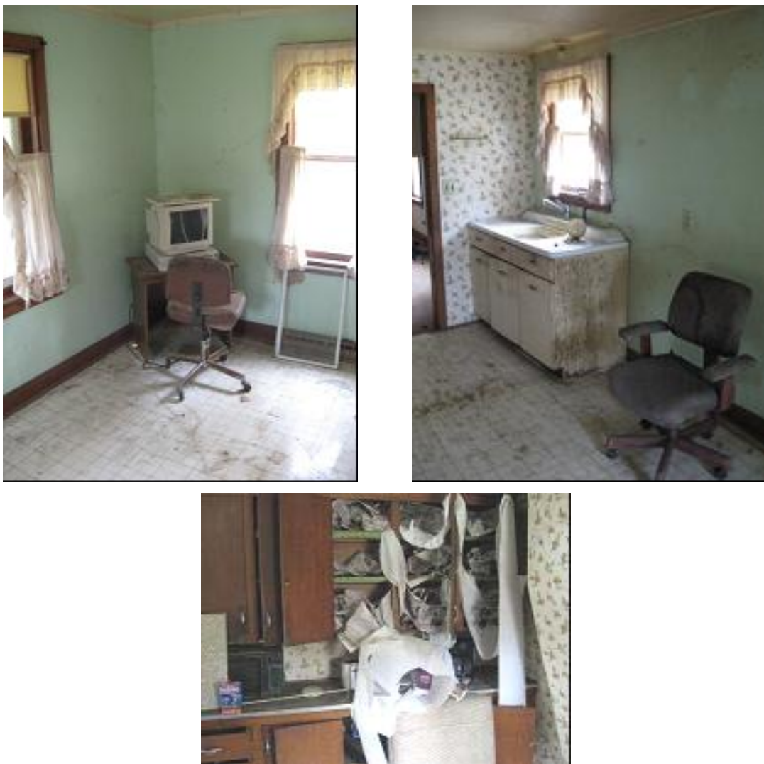
Figure 5-3: Kitchen prior to controlled field fire event. Kitchen ignition source is depicted in the bottom figure.
