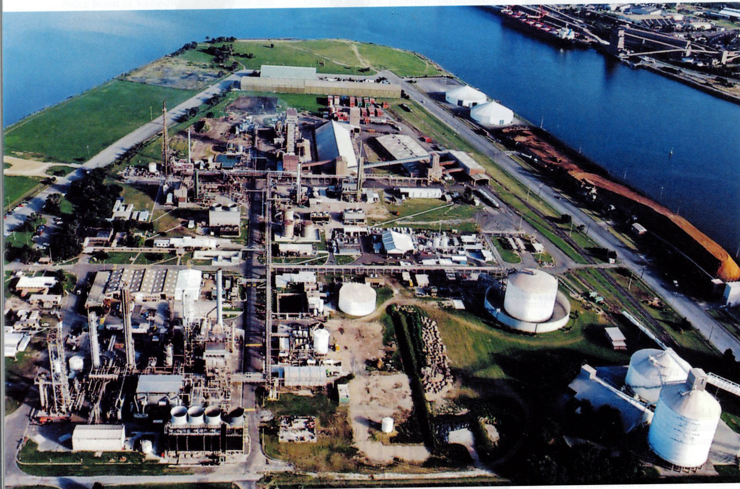
Orica's Kooragang Island plant.
