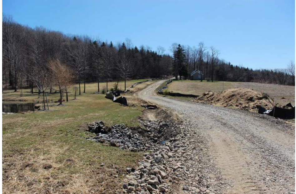
Photo 5.2 Nornew, Smyrna Hillbillies #2H, access road, Smyrna, Madison County NY. Photo taken during drilling phase of improved existing private dirt road (approximately 0.8 miles long). Not visible in photo is an additional 0.6 mile of new access road construction. Operator added ditches, drainage, gravel & silt fence to existing dirt road.
