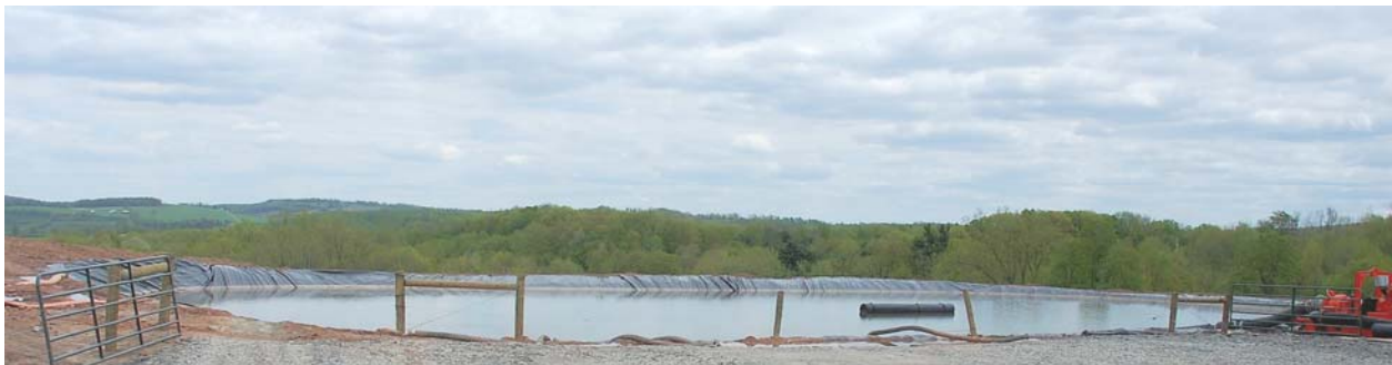
Photo 5.20 Fresh water supply pond. Black pipe in pond is a float to keep suction away from pond bottom liner. Ponds are completely enclosed by wire fence. Source: NYS DEC 2009.
