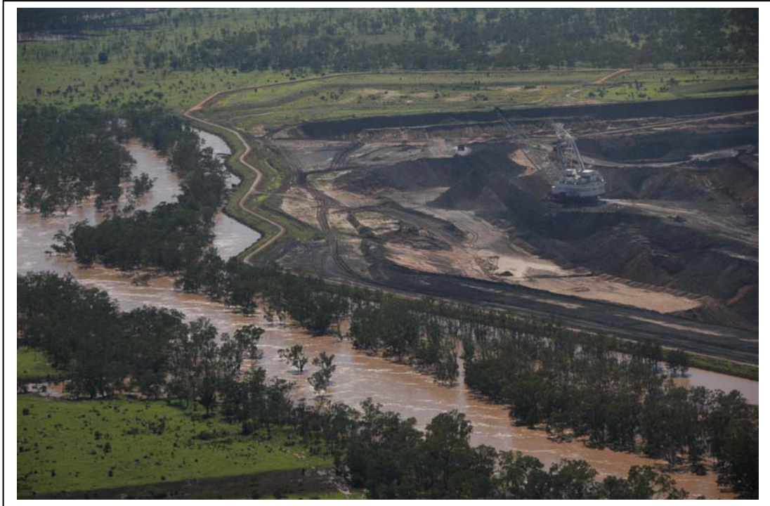
Curragh North. Levee is holding back Nogoa River <50km downstream of Ensham
