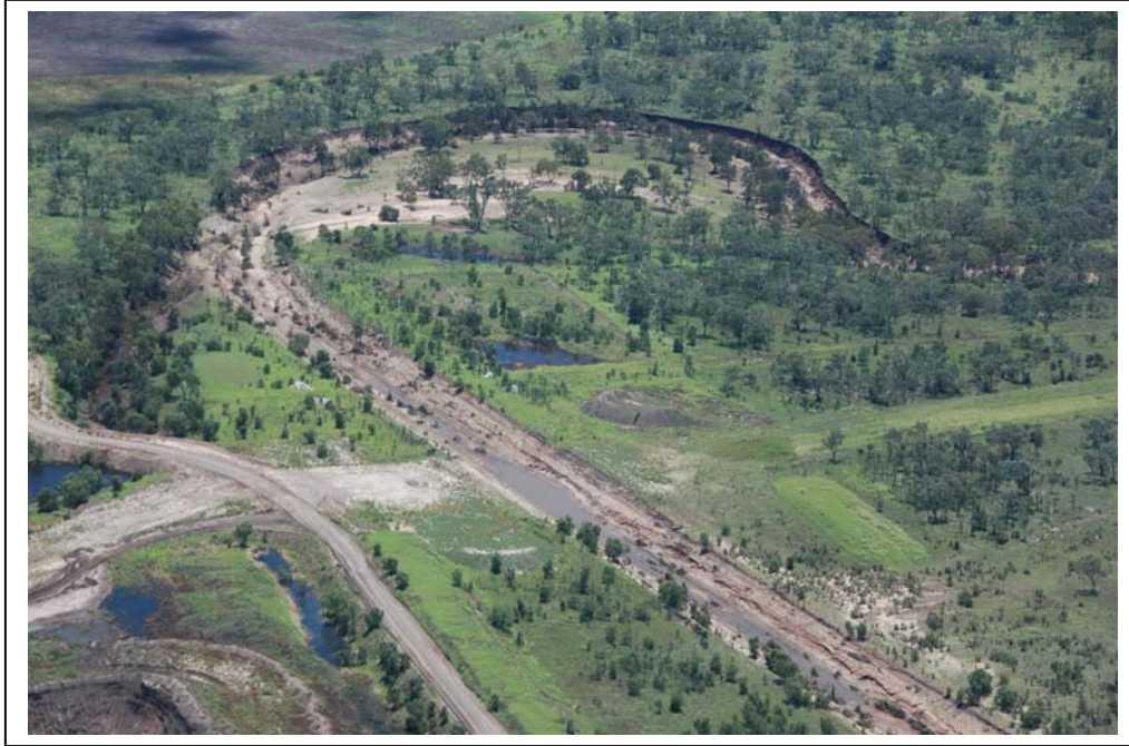
Stream Diversion – Stephen's Creek
