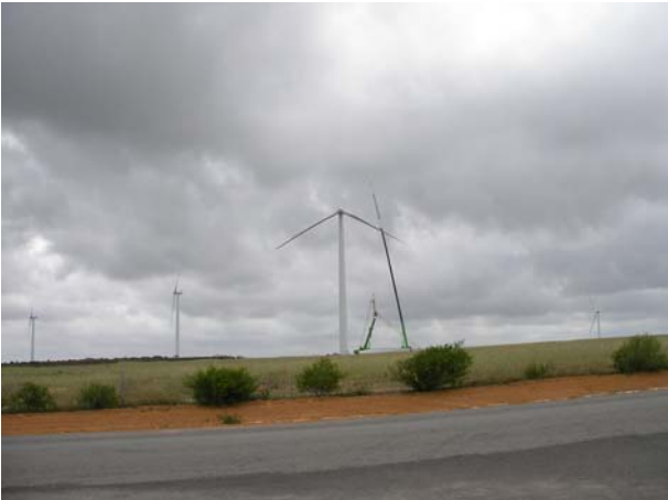
Crane repairing damaged turbine in Western Australia 2007.
