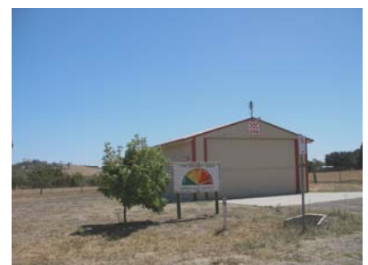
Tooborac Fire Station
