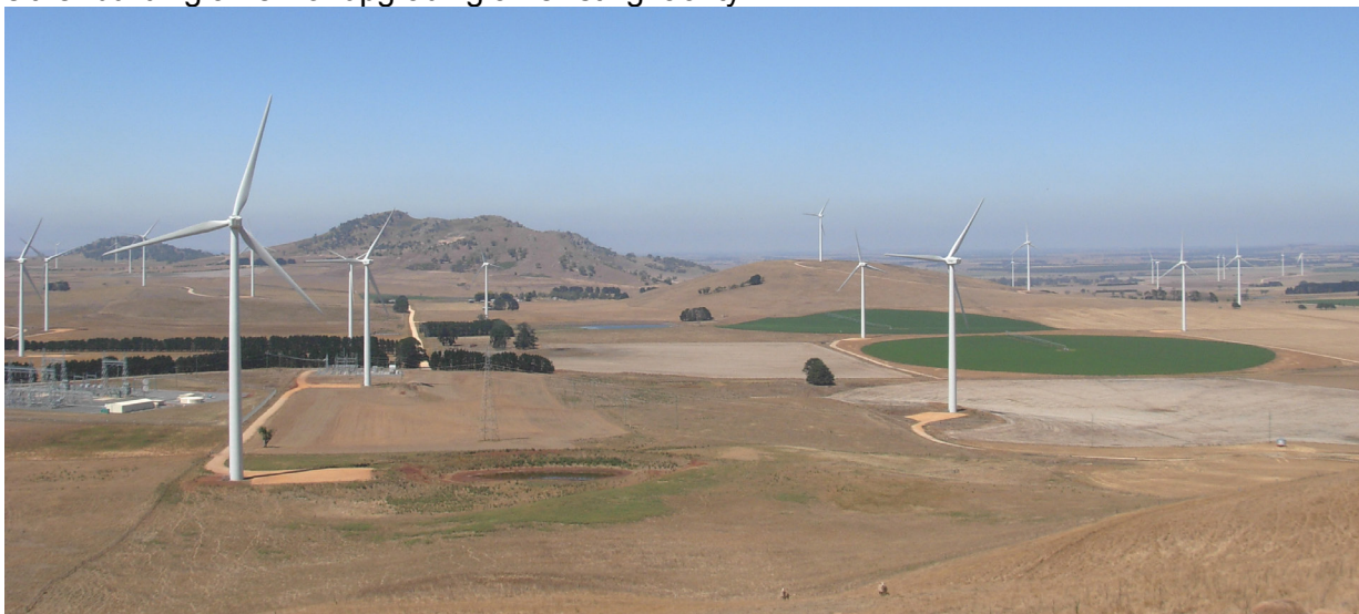
Wind energy facility in the landscape, including high voltage power lines and substations. Source: B. Gane.
