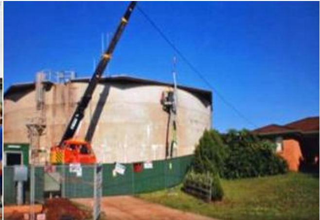
Image 5: Optus starting construction
