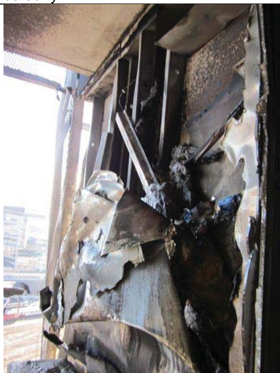
External wall at upper height
