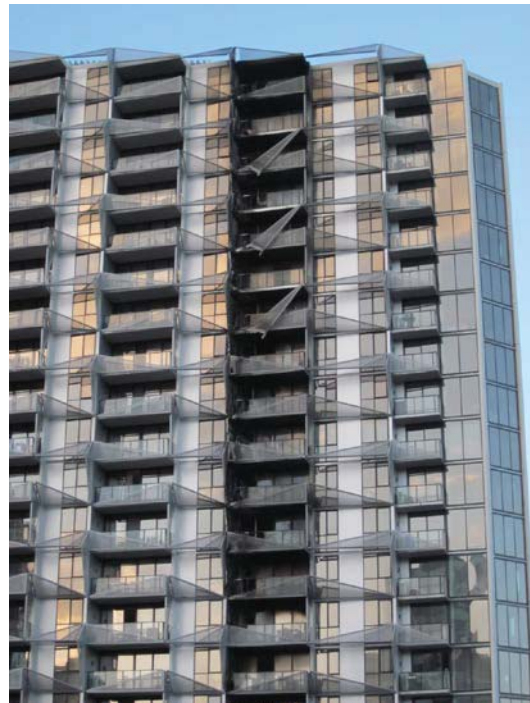
Photo Post Fire
