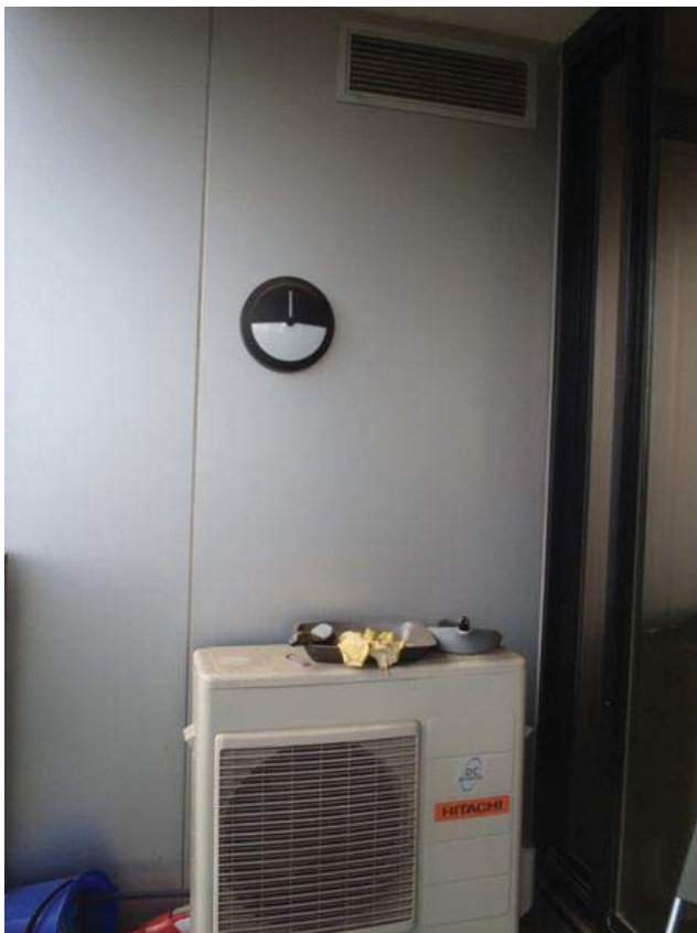
Figure 16 - Exhaust Grill Location, representative of all 05 Series Apartments.
