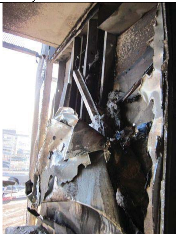
External wall at upper height
