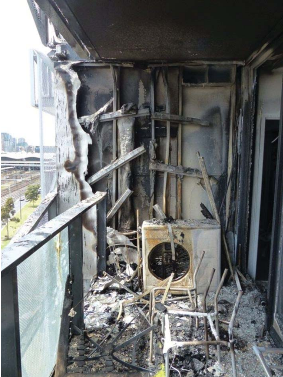
Figure 6 - Picture 5: South Wall Balcony of Apartment 805 before excavation.
