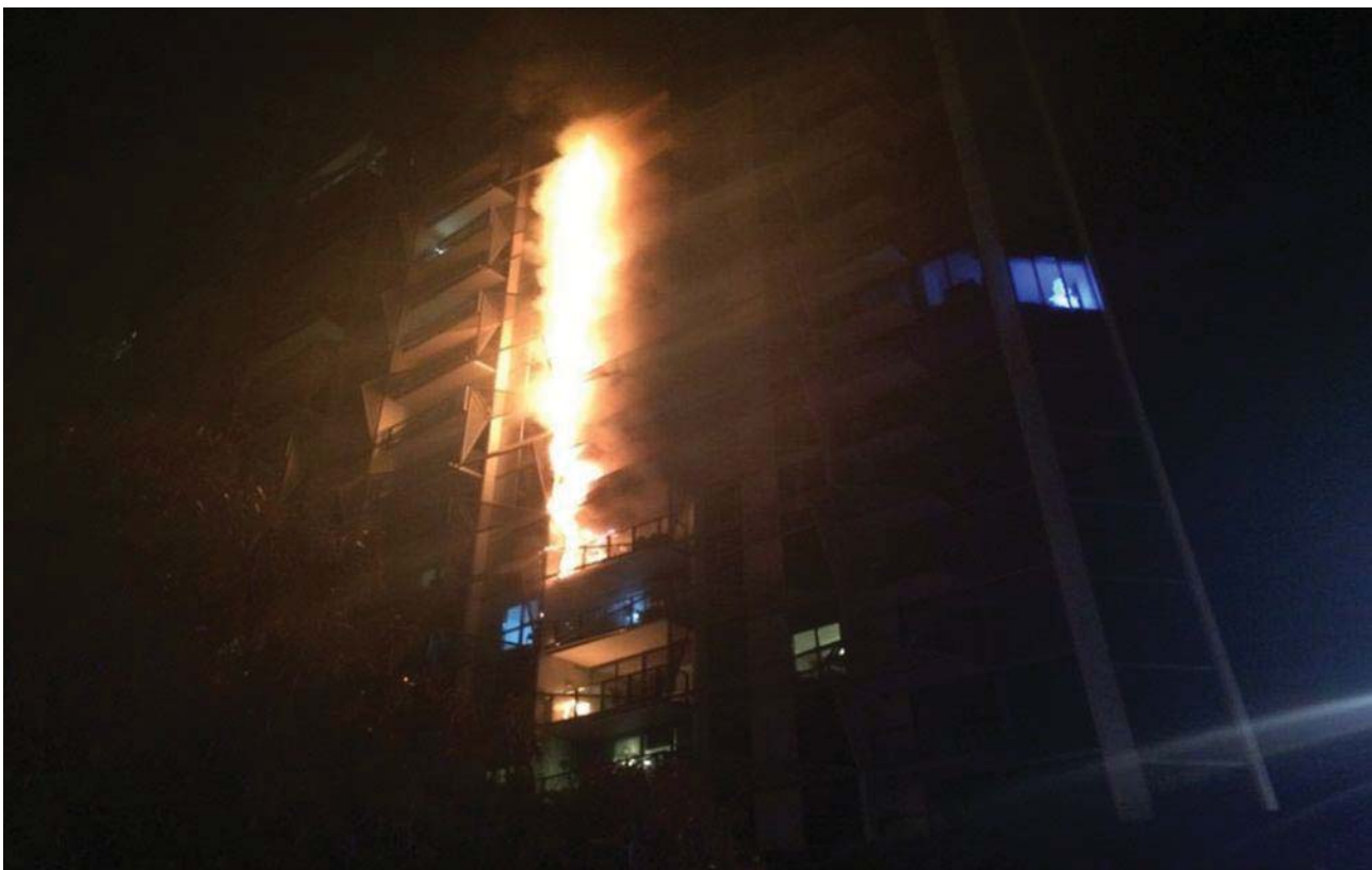
Figure 2 – Shows fire on level 6 and fire on level 8 (point of origin) extending up to level 14 (02:29)
