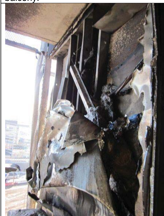
External wall at upper height
