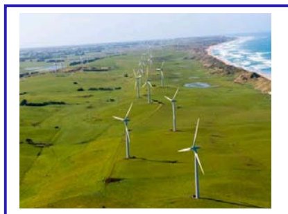
View of turbines at Codrington and Yambuk wind farm
