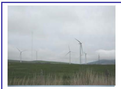
View of turbines at Waubra wind farm
