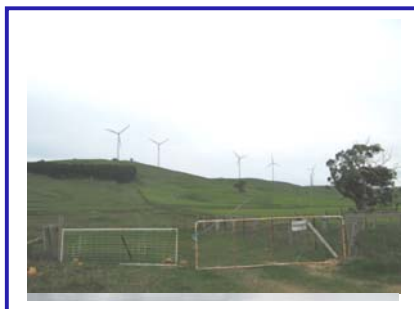
View of turbines at Challicum Hills wind farm from viewing area off Geelong Road
