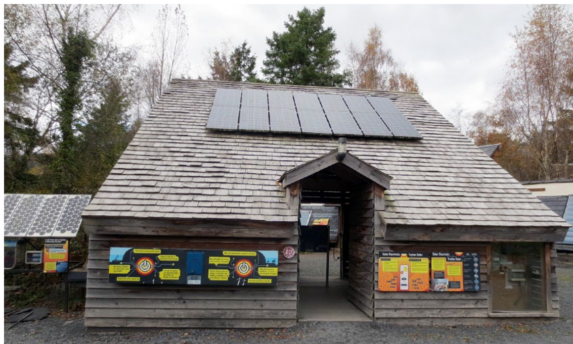
BUILDING SUSTAINABILITY: The Centre for Alternative Technology in Machynlleth, Wales.
