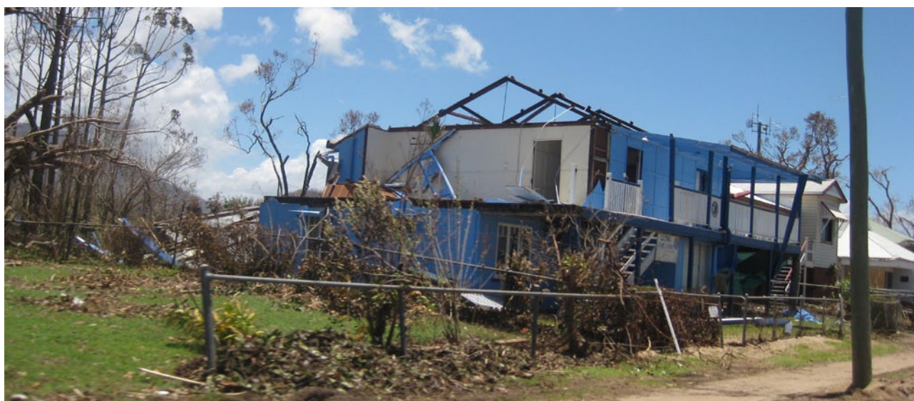
Photo: Cyclone Yasi damage, 2011.
