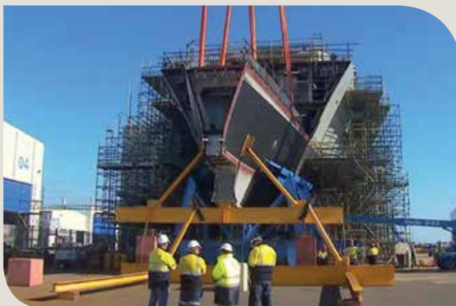
AWD under construction
