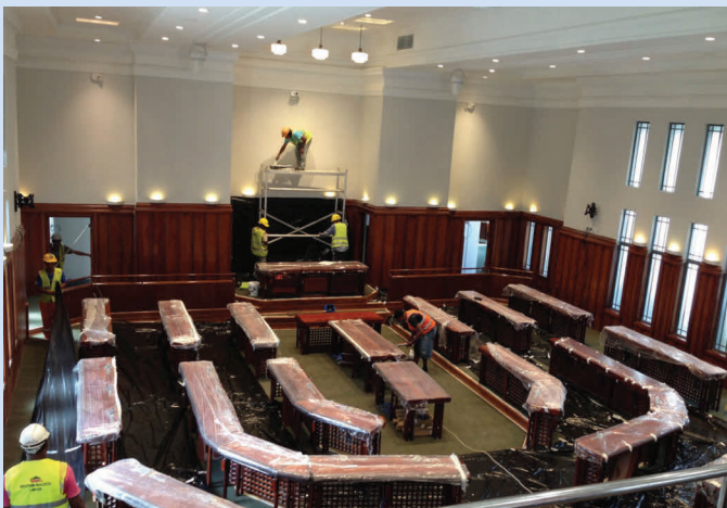
Restoration work on the chamber of the Parliament of Fiji.
